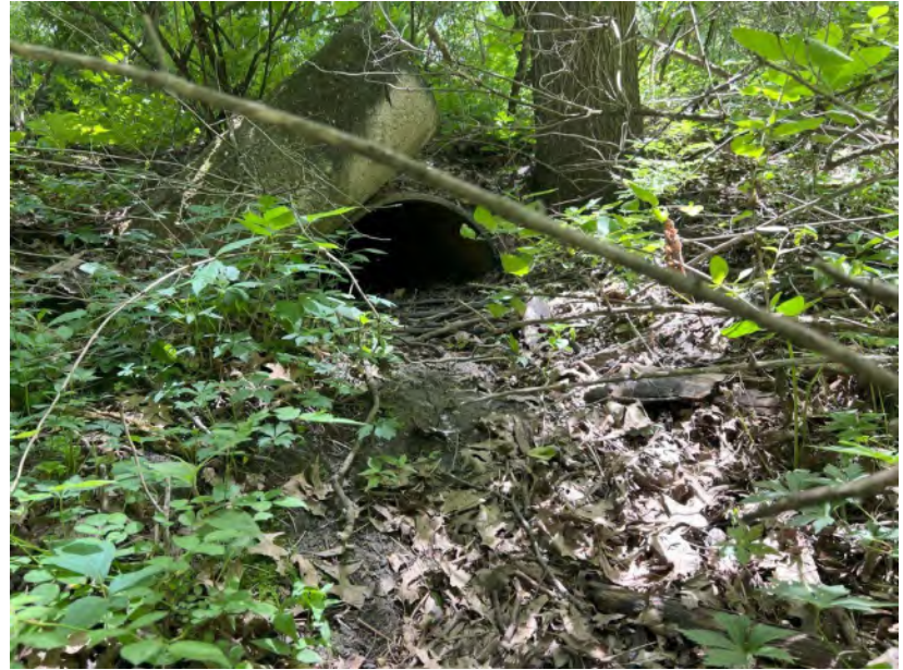
35. View south of culvert under the railroad. 6/6/2024.
